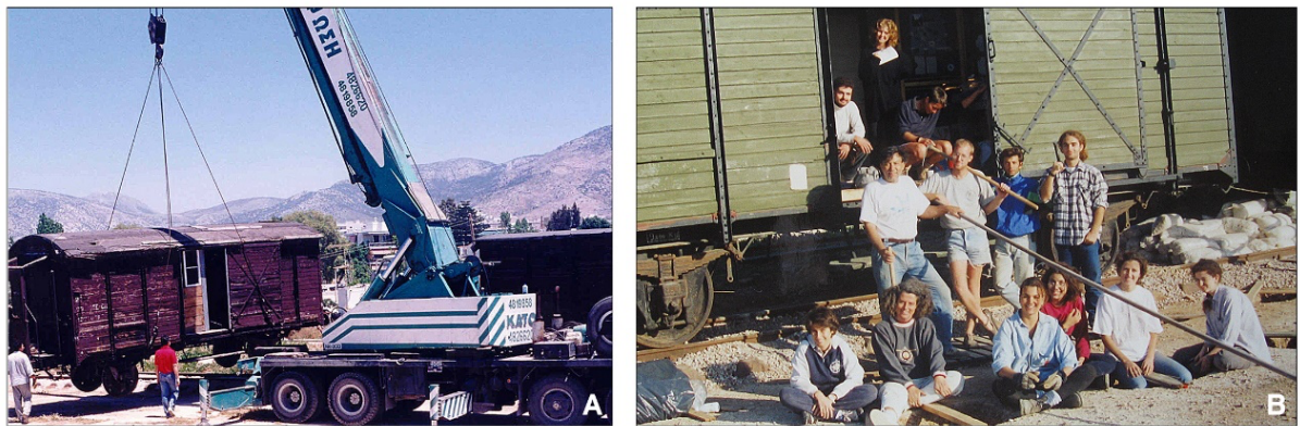
Figure 2. A: On 27 May 1994 two very old train wagons (weighing 12 tons each) were transported and mounted on rail track, which was installed previously. B: By November 1994 the two train wagons were almost fully renovated with help from ARCHELON members and volunteers.
